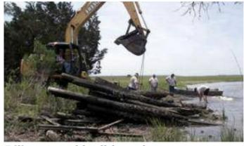
Pilings and bulkhead structures being removed to make way for the new Living Shoreline along Lawrence Creek at Cannon's Point.
